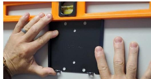
b) Ensure that the bracket is located adjacent to the wiring source (junction box) without impeding access to it.
